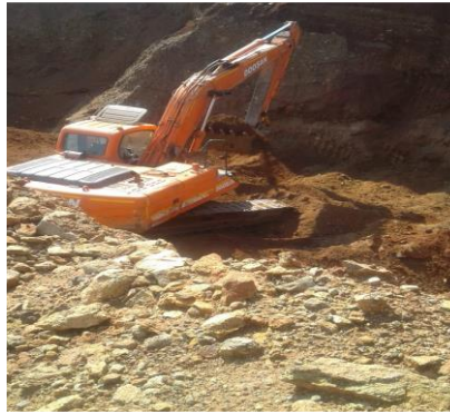
Figure 15: Mining operation of Chrome excavation by a hired Dozer, 2020
